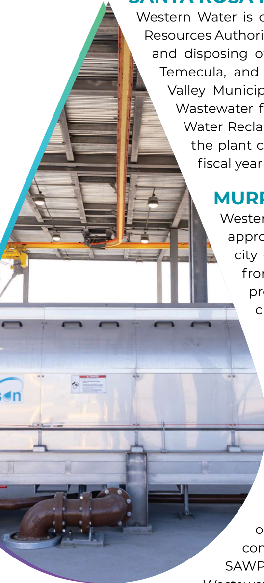
One of the rotary drum thickeners for wastewater at the Santa Rosa Regional Resources Authority (SRRRA)
