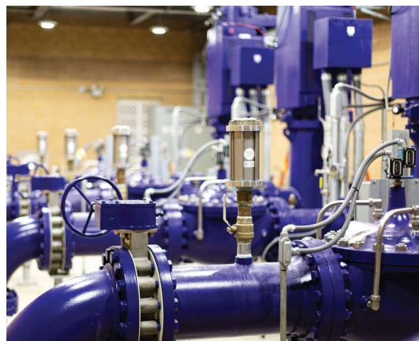
The Sterling Pump Station can pump more than 9,000 gallons of water per minute through the La Sierra Pipeline
