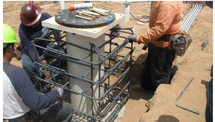
WBMWD Torrance Pump Concrete Pedestal
